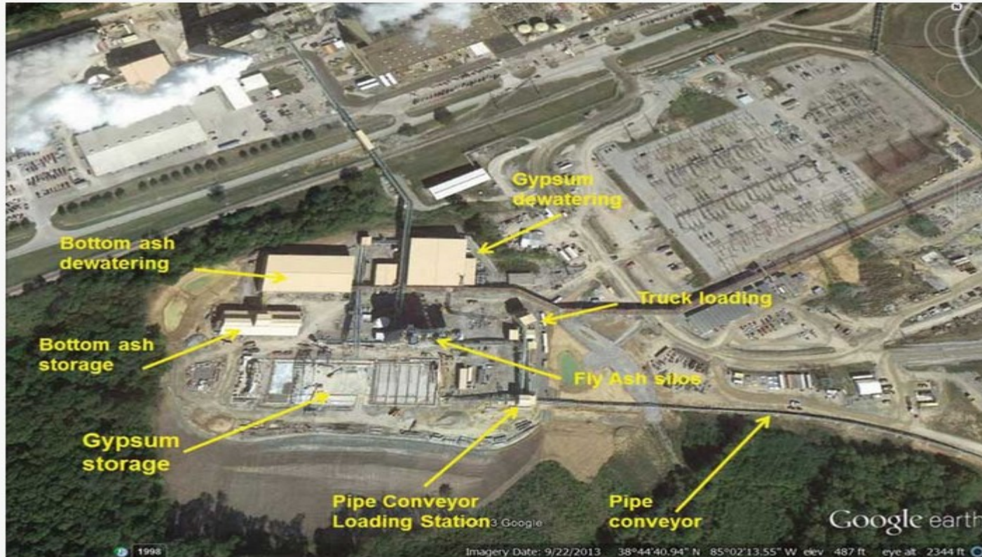
An aerial view of the Ghent CCR facility shows the scale of the project.
