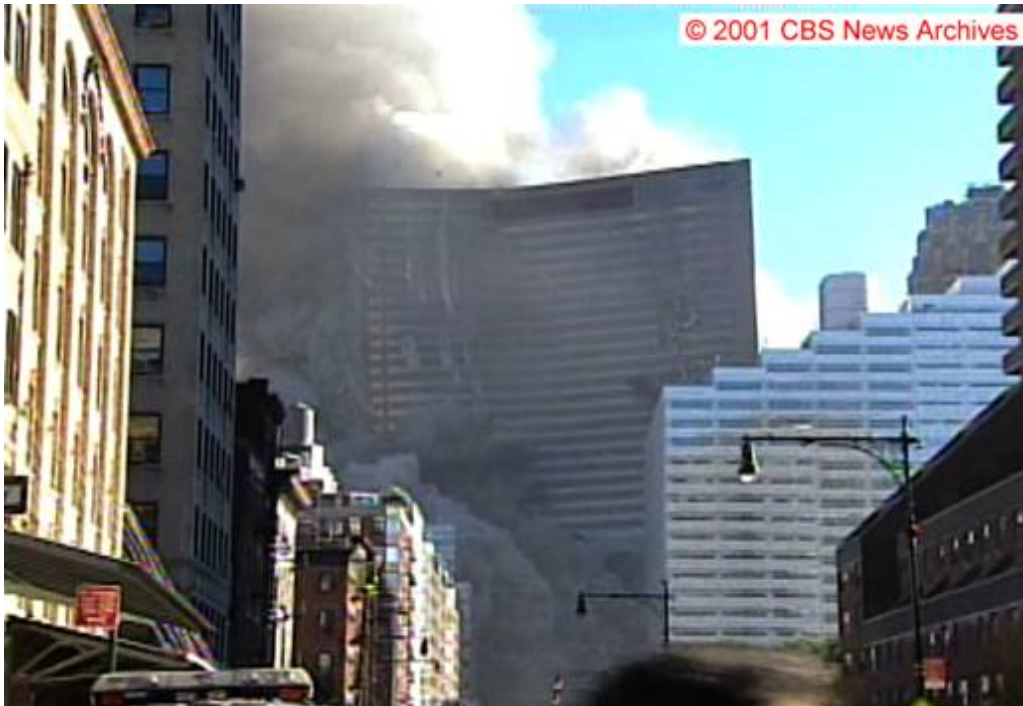
Figure 5–210. Frame from the Camera 9 video clip in Figure 5–192, showing the north face of WTC 7 10.0 \text{ s} \pm 0.2 \text{ s} after the east penthouse began to move downward. The intensities have been adjusted.
