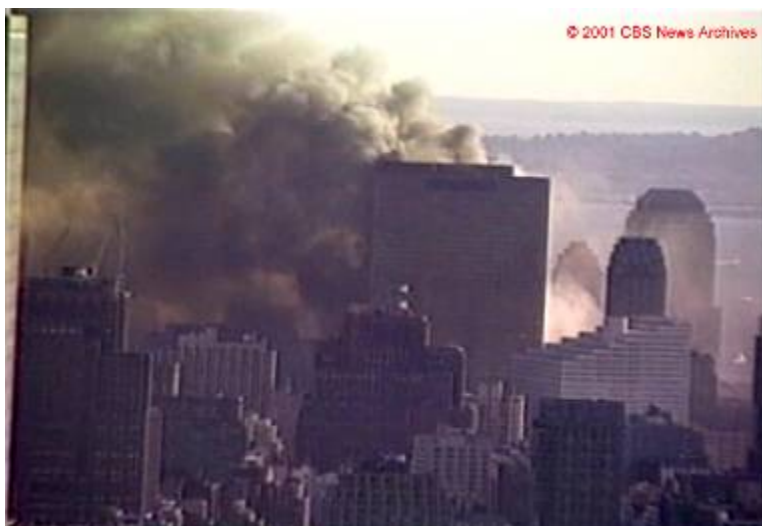
Figure 5-185. Frame from the Camera 2 video, showing the north face of WTC 7 (just right of center) seconds before the east penthouse began to fall into the building. The intensity levels were adjusted.
