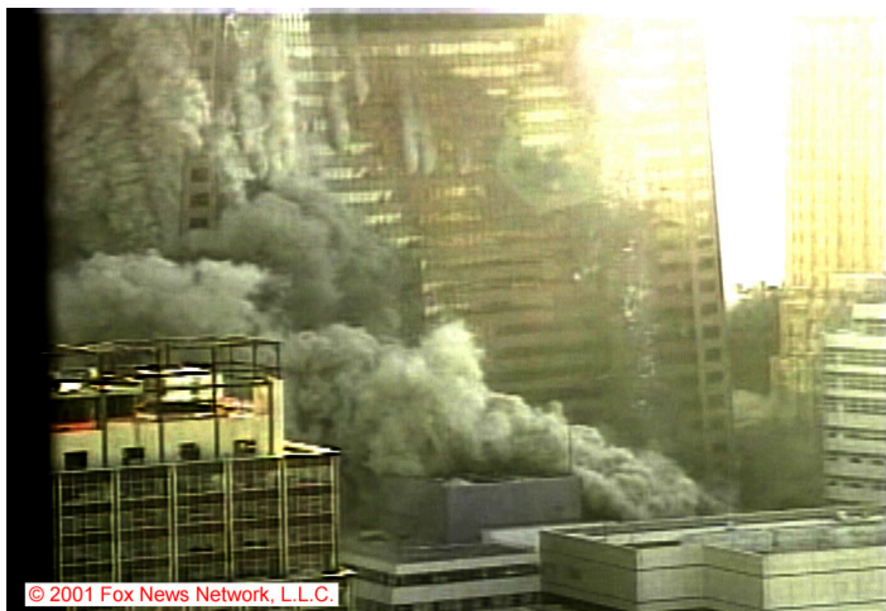
Figure 5–212. Frame from the Camera 6 video clip in Figure 5–189, showing the north face of WTC 7 11.0 \text{ s} \pm 0.2 \text{ s} after the east penthouse began to move downward. The intensities have been adjusted.
