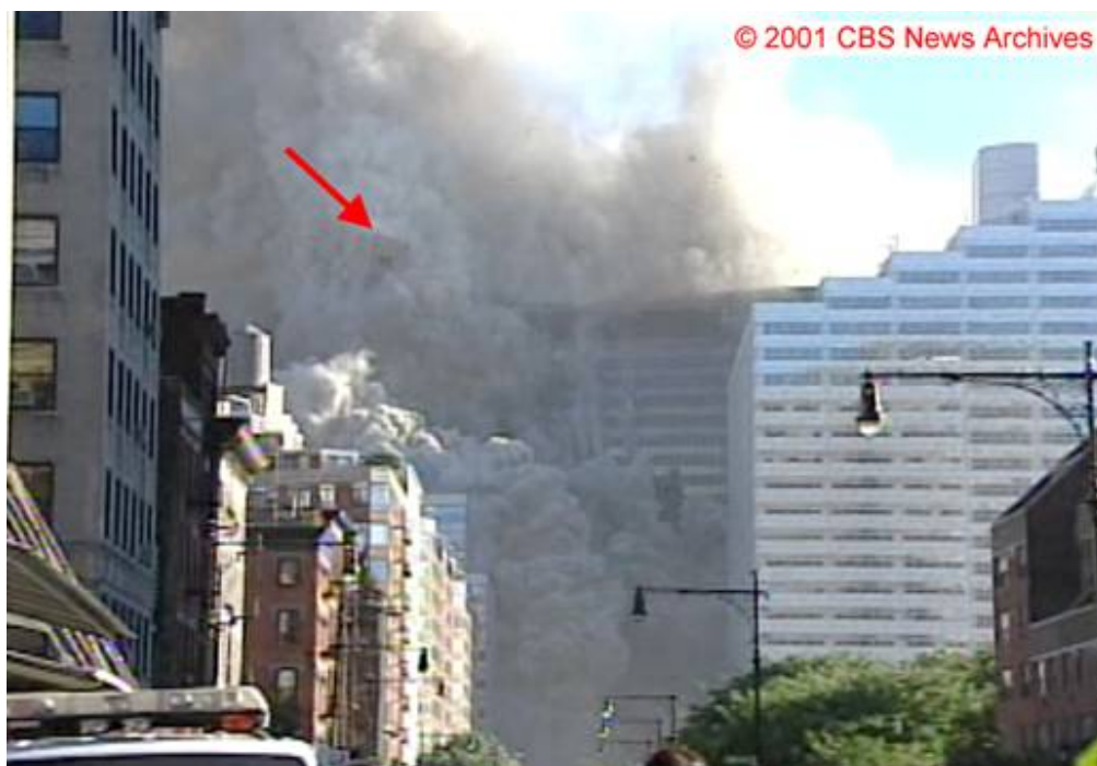
Figure 5-215. Frame from the Camera 9 video clip in Figure 5-192, showing the north face of WTC 7 12.0 \text{ s} \pm 0.2 \text{ s} after the east penthouse began to move downward.
