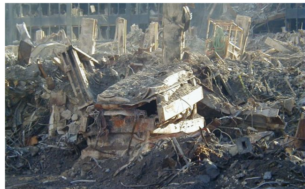
Figure A-7. Photographs taken on mid-October, 2001, showing Con Edison transformer #4 (or #8 or #9) uncovered from the debris pile of WTC 7.
