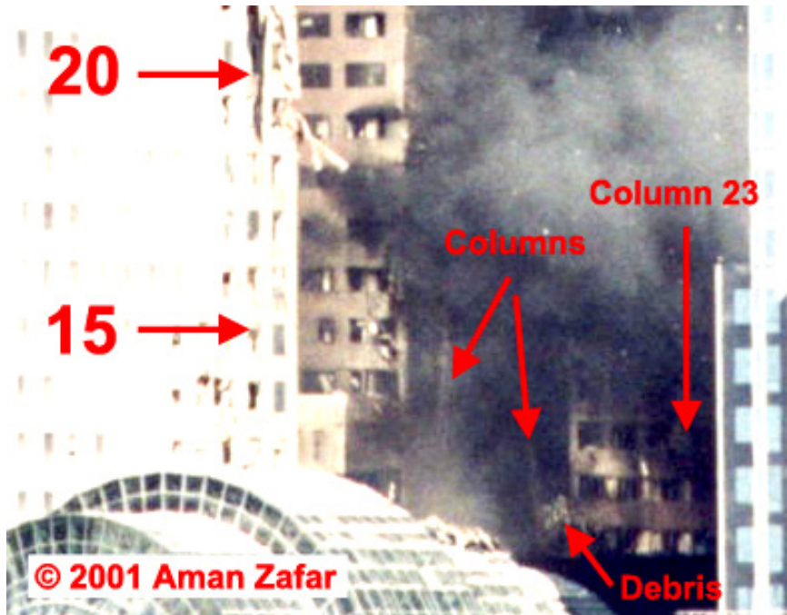
Figure 5-63. Enlargement of the lower part of the southwest corner of WTC 7 from Figure 5-62, with certain features identified. The intensity levels have been adjusted.
