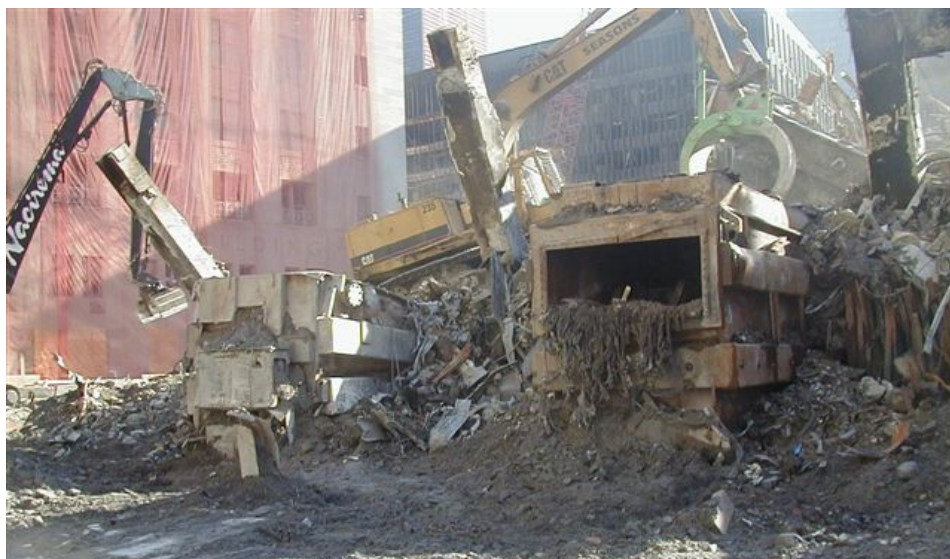
Figure A-8. Photograph taken in mid-October, 2001, showing Con Edison transformers #6 and #1 uncovered from debris pile of WTC 7.
