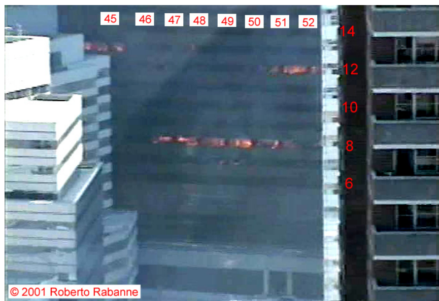
Figure 5–131. This frame from a video shot from a building to the northwest of WTC 7 was taken around 3:50:13 p.m. with an uncertainty of \pm 3 min. The intensities have been adjusted and column and floor numbers added.
