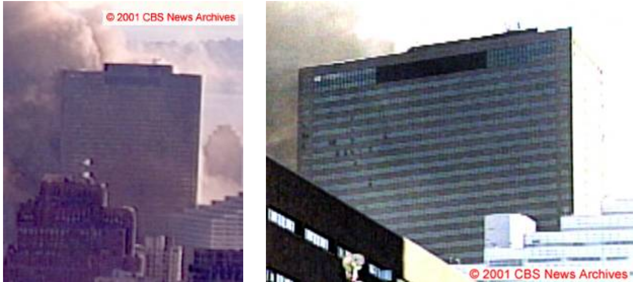
Figure 5–199. Cropped frames from the Camera 2 video clip in Figure 5–185 and the Camera 3 video clip in Figure 5–186, showing the north face of WTC 7 5.0 s \pm 0.1 s after the east penthouse began to move downward.
