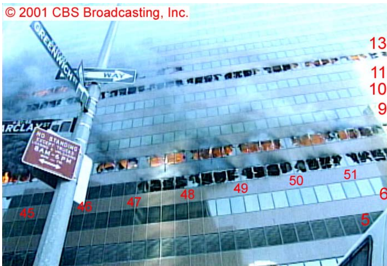
Figure 5–140. Frame taken from a video shot from near the corner of Greenwich and Barclay Streets showing the north face of WTC 7 between 3:51 p.m. and 3:58 p.m. The intensities have been adjusted, and column and floor numbers have been added.
