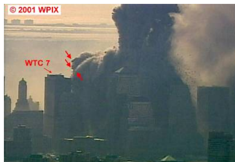
Figure 5–41. Three pairs of frames taken from videos shot from the north and west, showing the collapse of WTC 1. Times are relative to the start of the collapse. Arrows indicate large objects that were projected toward WTC 7. The intensities of the video frames have been adjusted.
