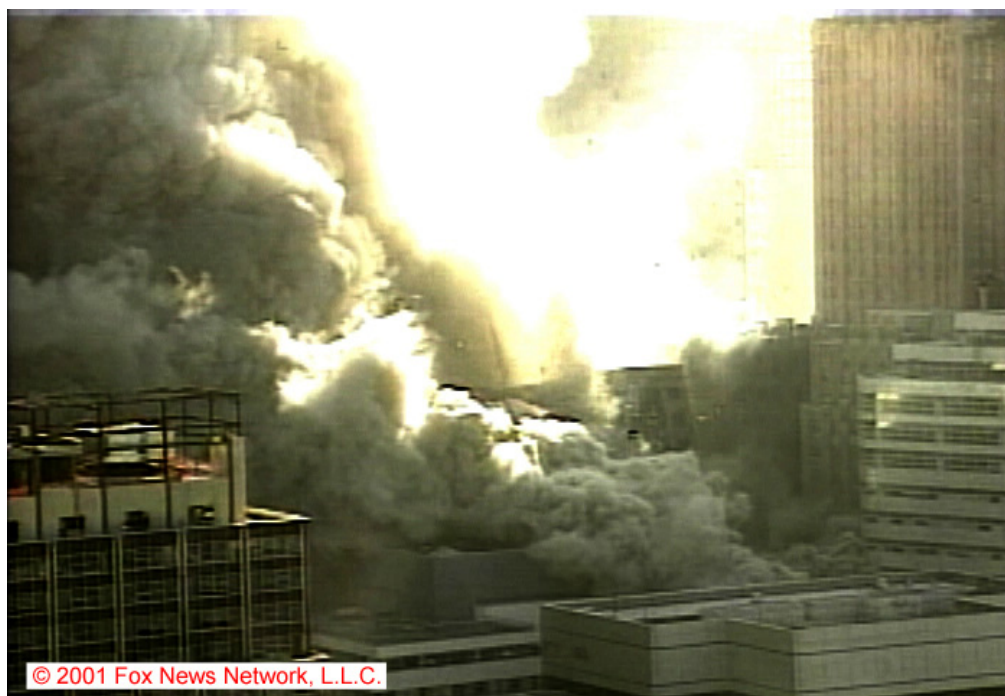
Figure 5-216. Frame from the Camera 6 video clip in Figure 5-189, showing the north face of WTC 7 13.0 \text{ s} \pm 0.2 \text{ s} after the east penthouse began to move downward.
