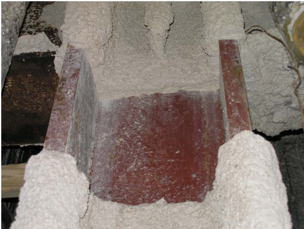
Figure 2-35. Column with removed SFRM and intact primer.
