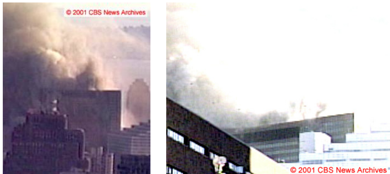
Figure 5–211. Cropped frames from the Camera 2 video clip in Figure 5–185 and the Camera 3 video clip in Figure 5–186, showing the north face of WTC 7 11.0 \text{ s} \pm 0.1 \text{ s} after the east penthouse began to move downward. The intensities have been adjusted.
