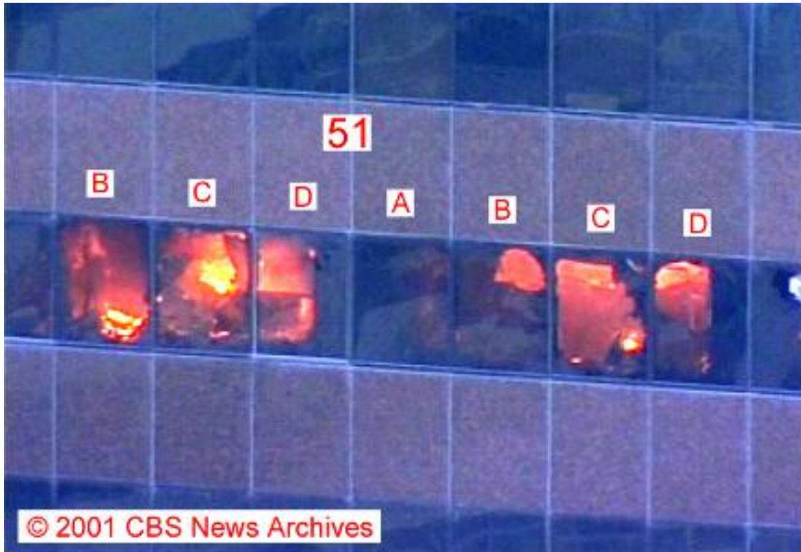
Figure 5-120. Frame taken from a video clip shot looking down on WTC 7 from a building to the northwest showing the fires along a length of the north side of the 7 th floor of WTC 7.
