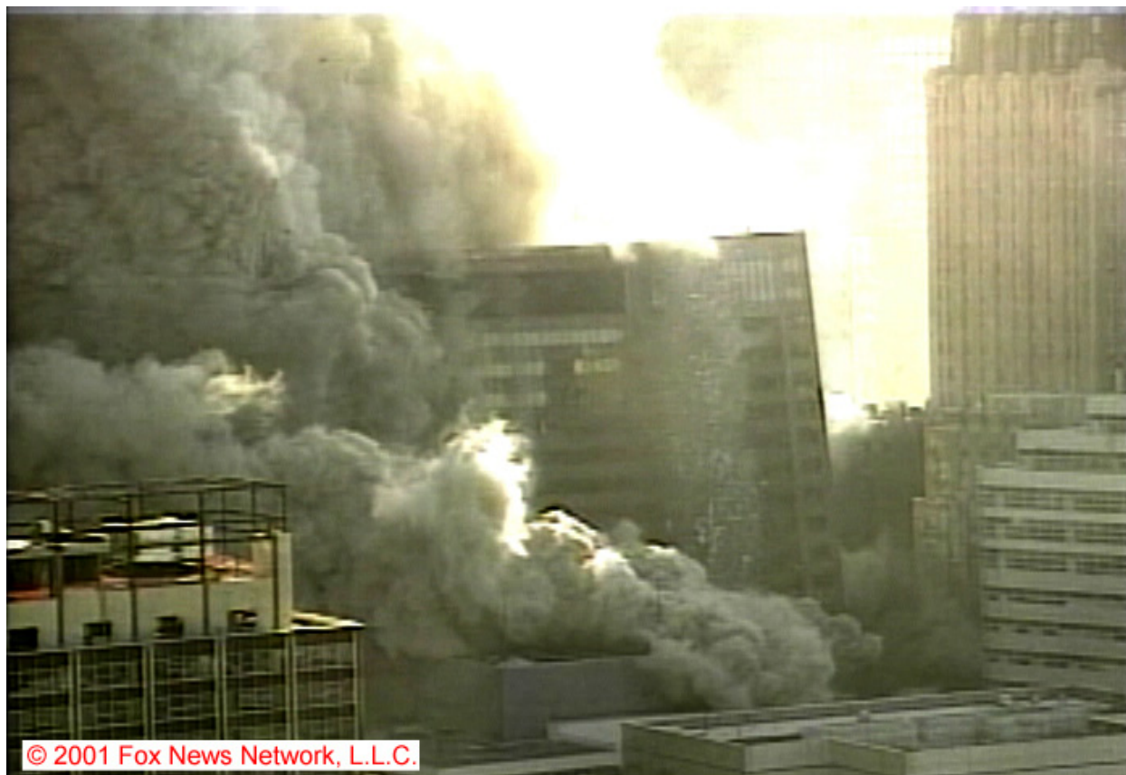
Figure 5–214. Frame from the Camera 6 video clip in Figure 5–189, showing the north face of WTC 7 12.0 s \pm 0.2 s after the east penthouse began to move downward.
