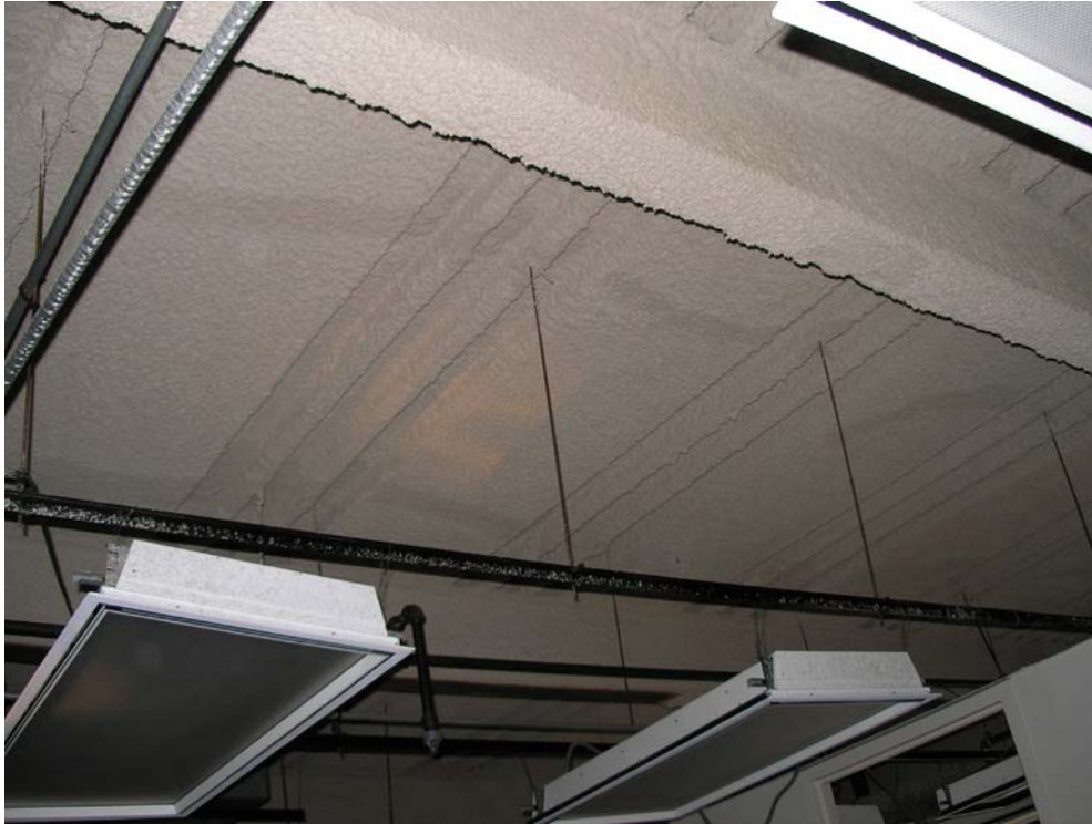
Figure 2-34. Floor beams with intact SFRM.
