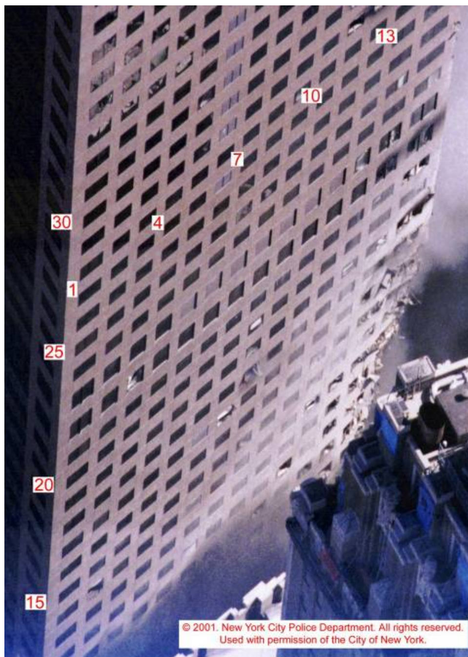
Figure 5–86. Image, cropped from Figure 5–67, showing the west face of WTC 7, shot from a helicopter between 2:30 p.m. and 3:00 p.m. Column and floor numbers have been added.
