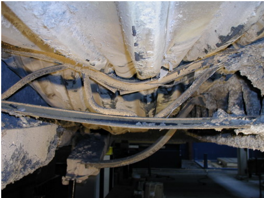
Figure 5–70. View looking north of south bridging truss at location where concrete spalling occurred on Assembly 4.
