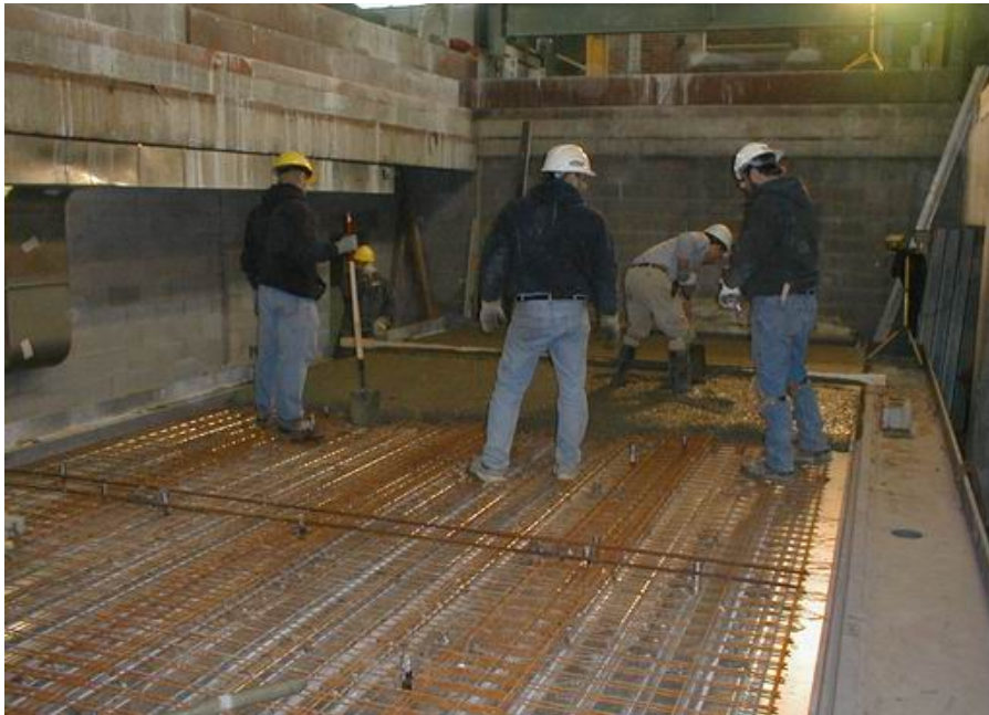
Figure 4–17. Concrete placement.
