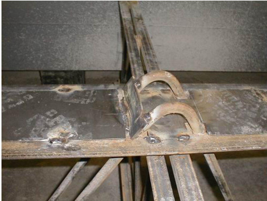
Figure 4–11. Cover plates on main truss.
