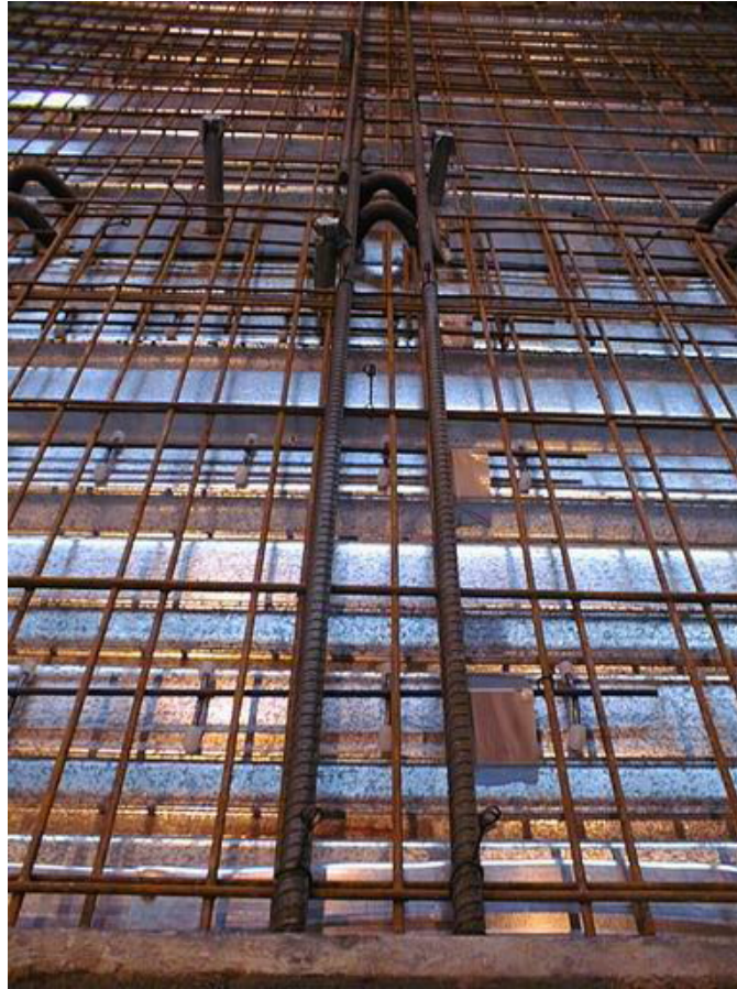
Figure 4–29. Welded wire fabric and rebar.
