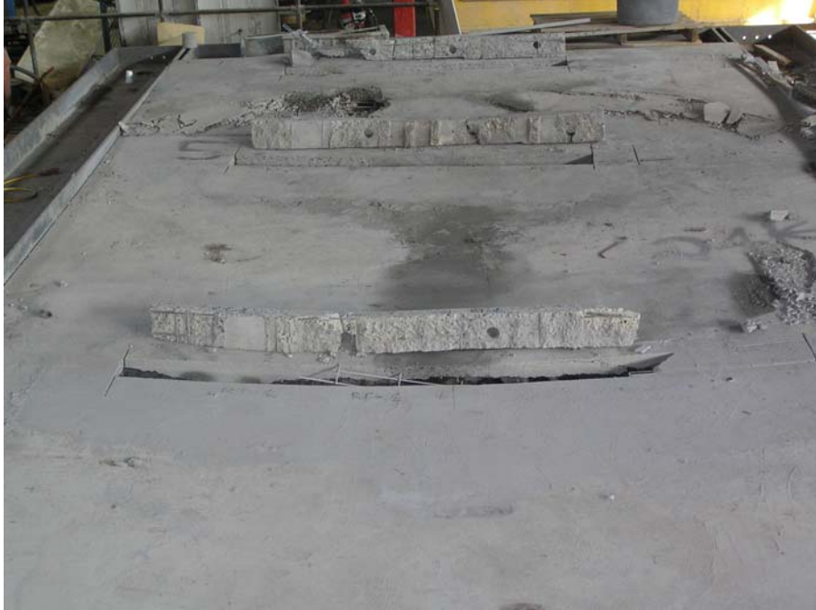
Figure 5–20. Sections cut through concrete slab to confirm delamination spalling.
