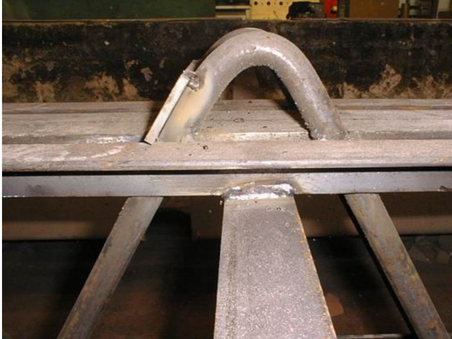
Figure 4-24. Intersection of main truss and deck support angle.
