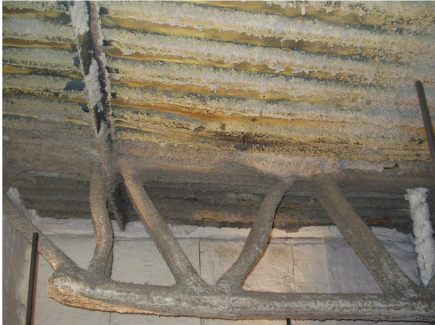
Figure 5–35. View of core end diagonal strut of north main truss on Assembly No. 2.
