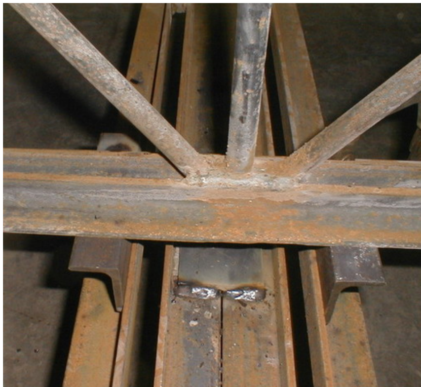
Figure 4–12. Intersection of main and bridging truss, bottom chord.
