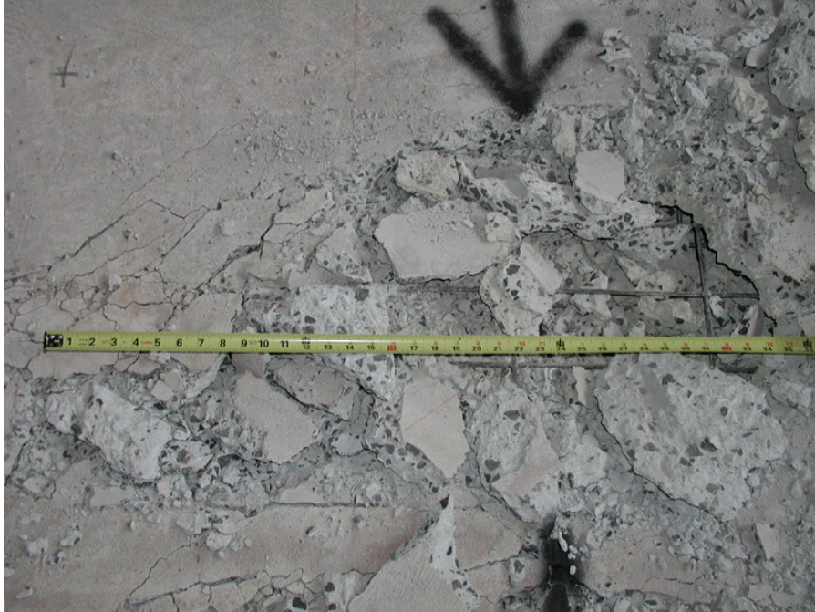
Figure 5–16. Close-up of spalling concrete at east end of Assembly No. 1.
