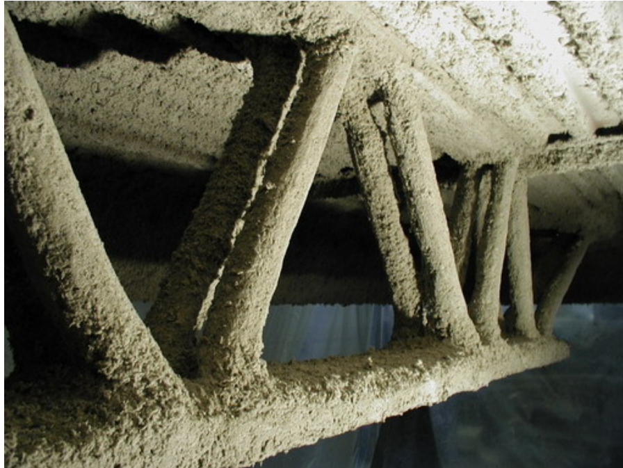
Figure 4-21. SFRM on main truss.
