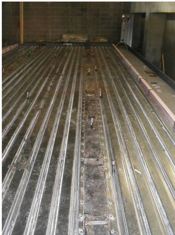
Figure 4–14. Placement of steel form deck.
