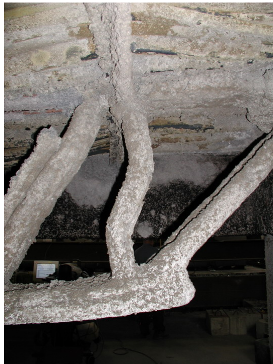
Figure 5–19. View of core-end diagonal strut of south main truss on Assembly No. 1.
