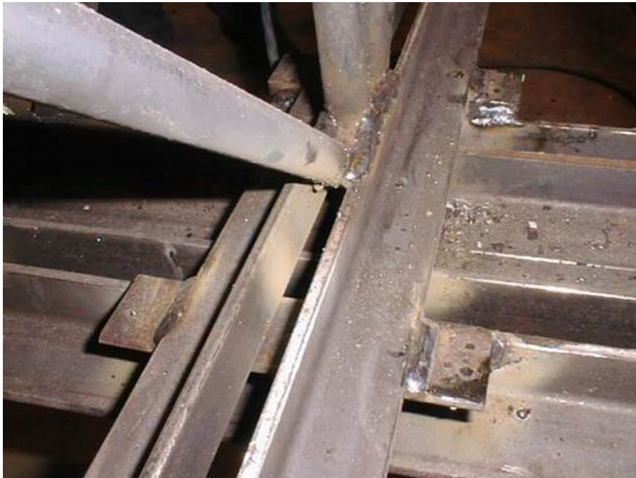
Figure 4-25. Intersection of main and bridging truss bottom chord.
