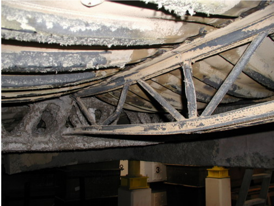
Figure 5–69. Intersection of north bridging and west main truss on Assembly 4.
