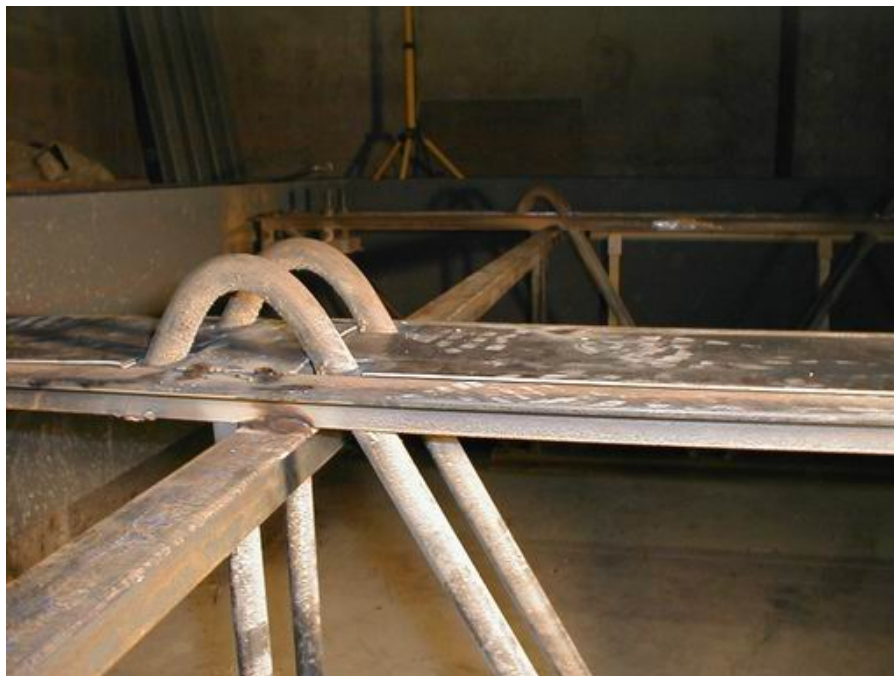
Figure 4–10. Intersection of deck support angle and main truss.
