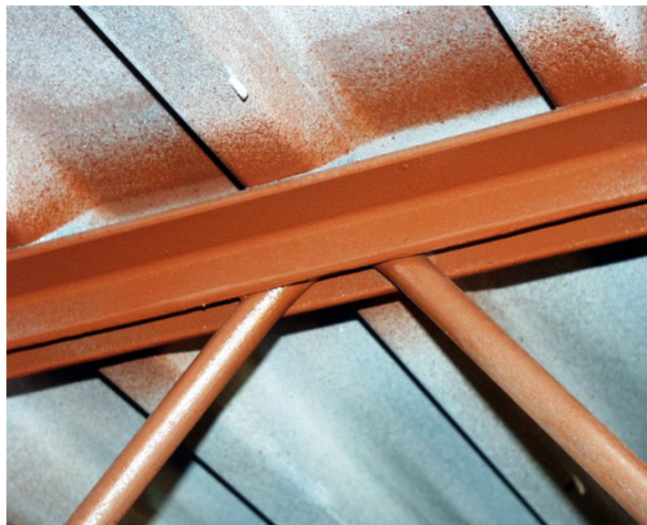
Figure 4–19. Primer on bridging truss.
