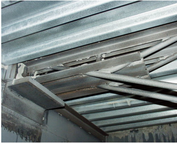
Figure 4–18. Sandblasted assembly.
