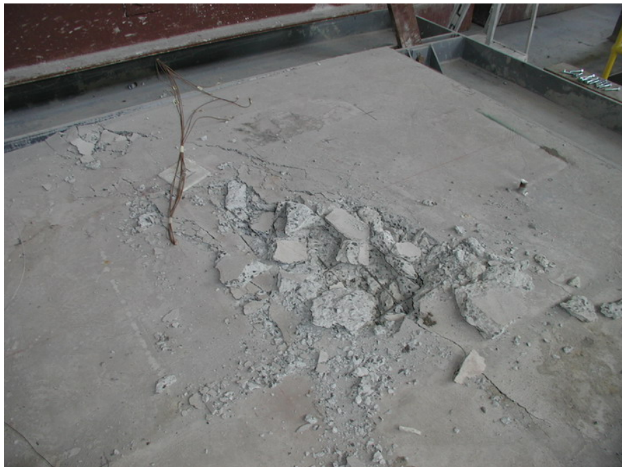
Figure 5–15. Detail of spalling concrete at east end of Assembly No. 1.
