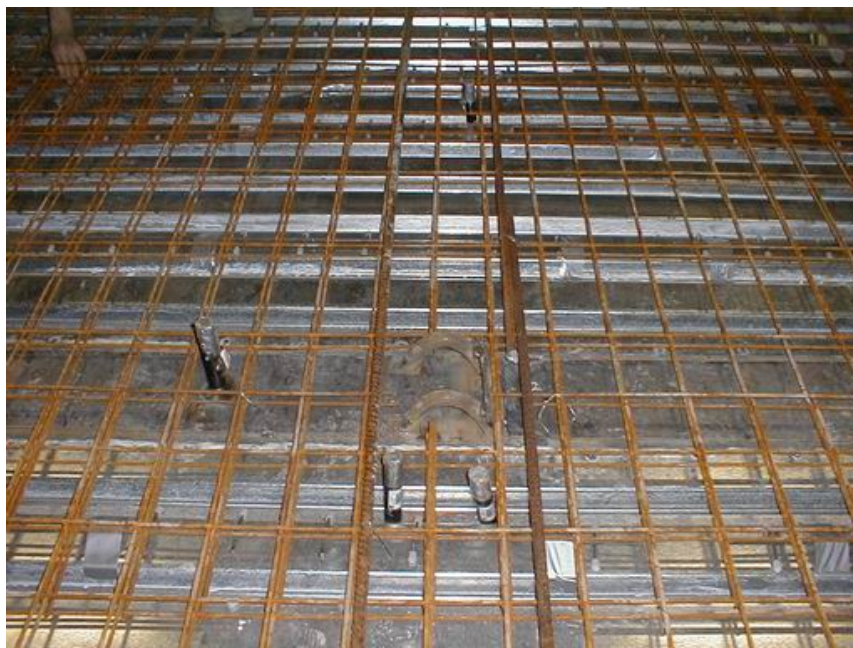
Figure 4–16. Welded wire fabric.
