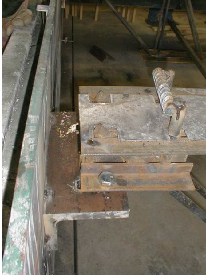
Figure 4–13. Detail of rebar welded to end stiffener.
