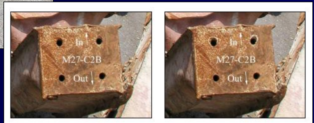
Figure 3-47, NCSTAR1-3C Perimeter column from WTC 1 Floor 92
